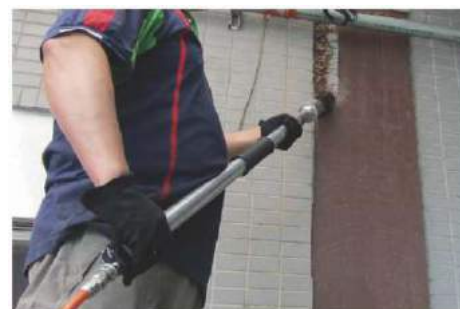
Corrosion removal for inaccessible area
